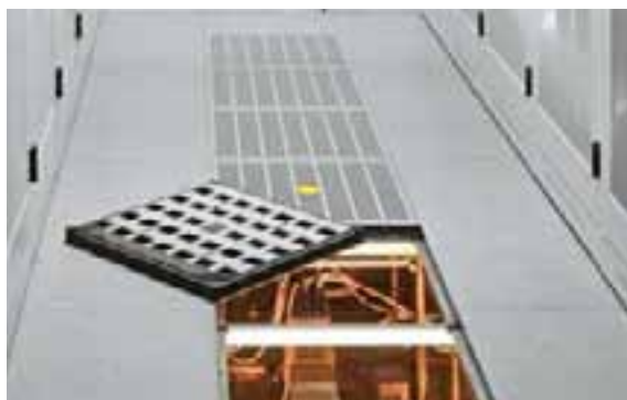
Power station, Unterföhring
